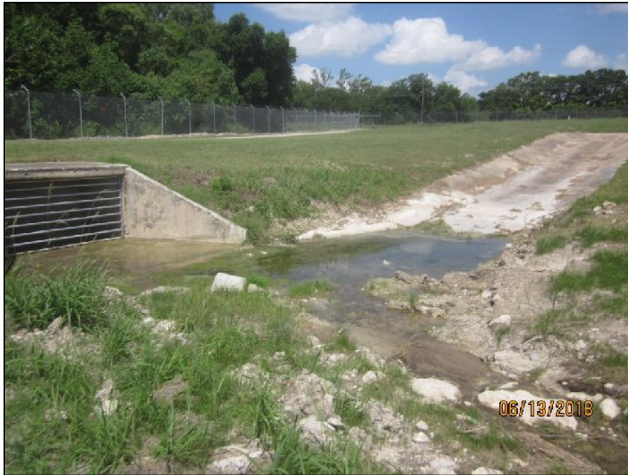
Photograph 7. View of the outfall at the downstream end of the wetland. Water was observed seeping from the soils in this area.
