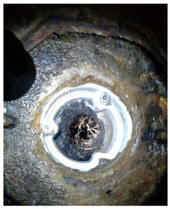
**Bathhouse Men's Changing Area:** An example of the failure of a sanitary sewer line in the Mens' Changing Area restrooms. Much of the existing plumbing within the Bathhouse is seventy years old and in poor physical condition.
