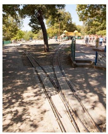
**Zilker Zephyr:** The Zilker Zephyr has been in service since the early 1960s. The track, which is visibly irregular and variable in gauge, appears to be approaching the end of its serviceable lifespan.
