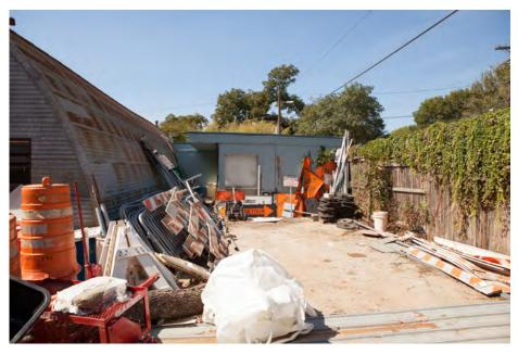
Maintenance Yard: The Quonset storage building, although an interesting structure, has reached a serviceability limit state. The extent of rust visible on the exterior of the building, and the number of open holes visible from the interior, indicate a building past economic rehabilitation. It would be less expensive to replace this building than it would to repair it for a different use.
