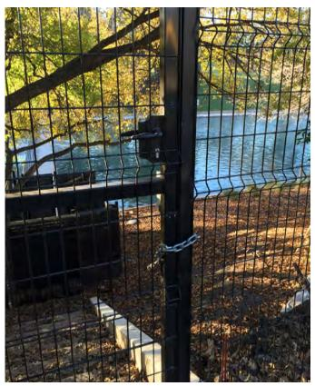
**Pool Enclosure:** Emergency egress from the pool enclosure is a matter of significant concern. Exits from the enclosure do not comply with current code requirements, a deficiency compounded by features such as locked gates.
