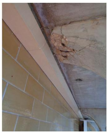
**Bathhouse Men's Changing Area:** The concrete canopy structures in the mens' and womens' changing areas are in poor condition, with a significant percentage exhibiting spalling concrete and exposed reinforcing.
